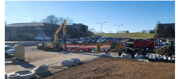
Hopewell East Construction Photo
